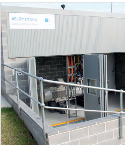
High-output BK 52 blocks supply CNG to vehicles in Sydney's public transport network.
